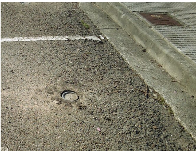
Figure 19: Image of a mote installed in a perpendicular parking lot
